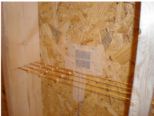
Figure 1. Instrumentation of the test wall cavity.
