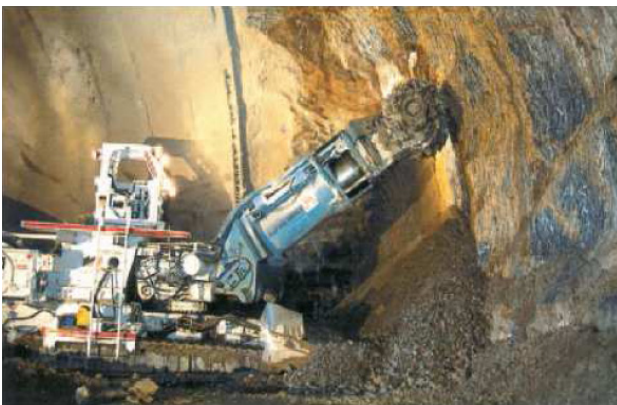
Fig 1. Rock excavation with a roadheader
