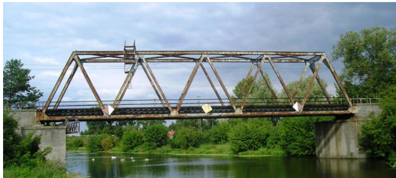
Fig. 1 Investigated railway truss bridge in Nieporet
