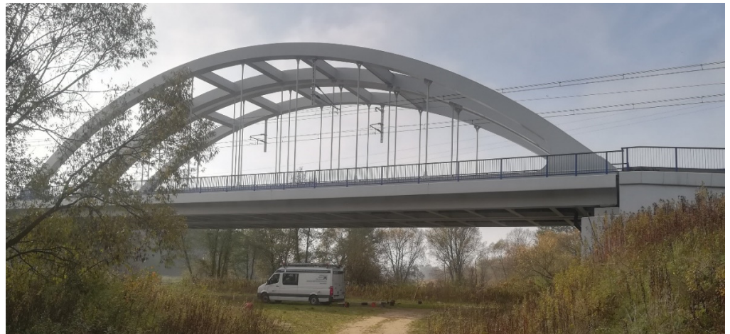
Figure 7. View of bridge No 2.
