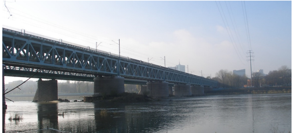
Figure 4. View of bridge No. 1.
