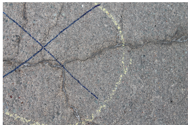
FIGURE 1. Surface cracking of concrete highway pavement suspected to be due to ASR.
