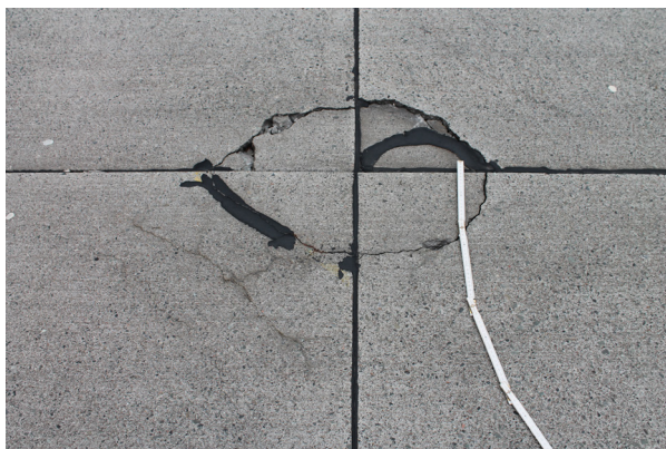
FIGURE 1. Surface cracking of concrete highway pavement suspected to be due to ASR.
