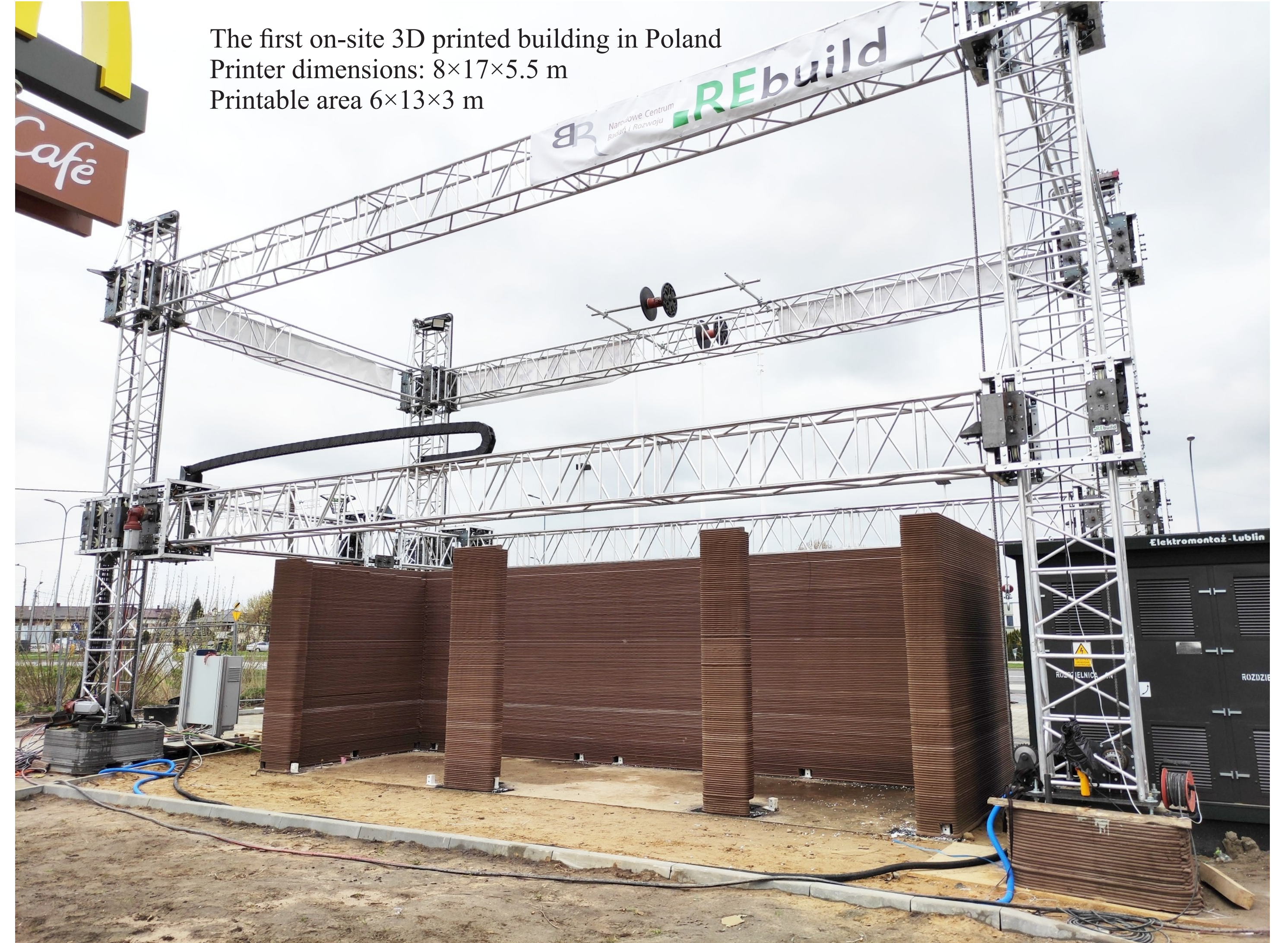
An industrial 3D printer with a workspace of 15/5/5 m, capable of printing with concrete or extruded polystyrene and milling.
